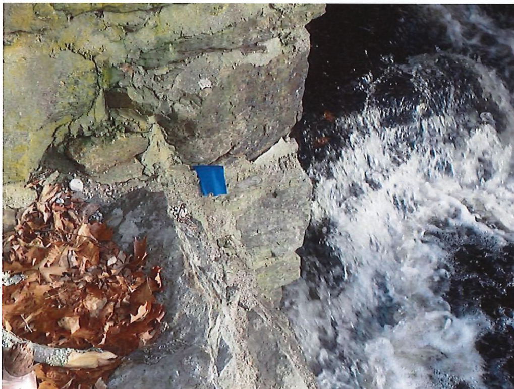
Photo 14: Cracked stone to the Northwest wingwall and breastwall interface.
