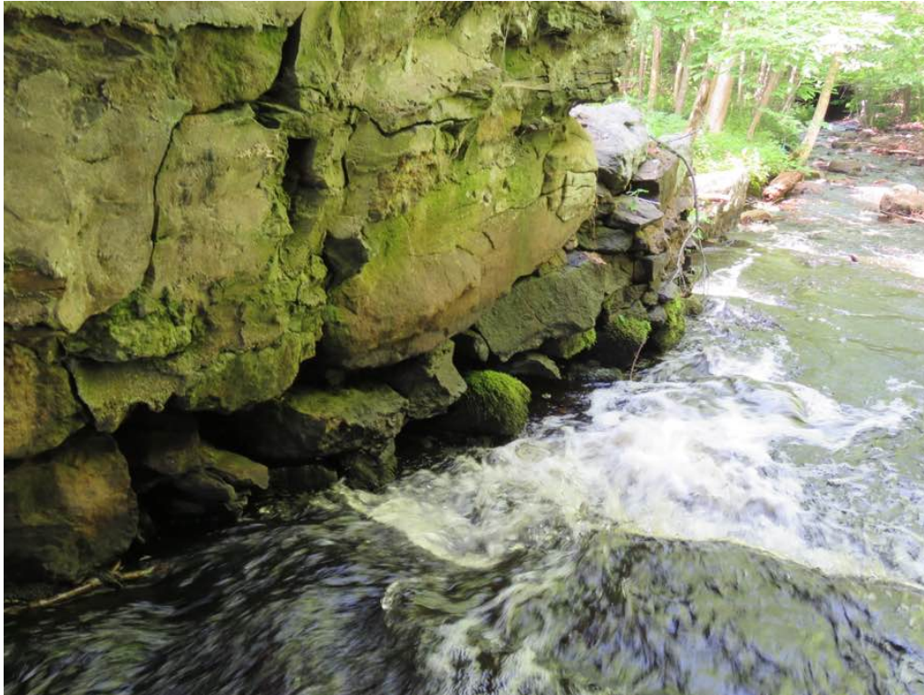
Photo 5: South breastwall, West end, voids to the bottom stones.
