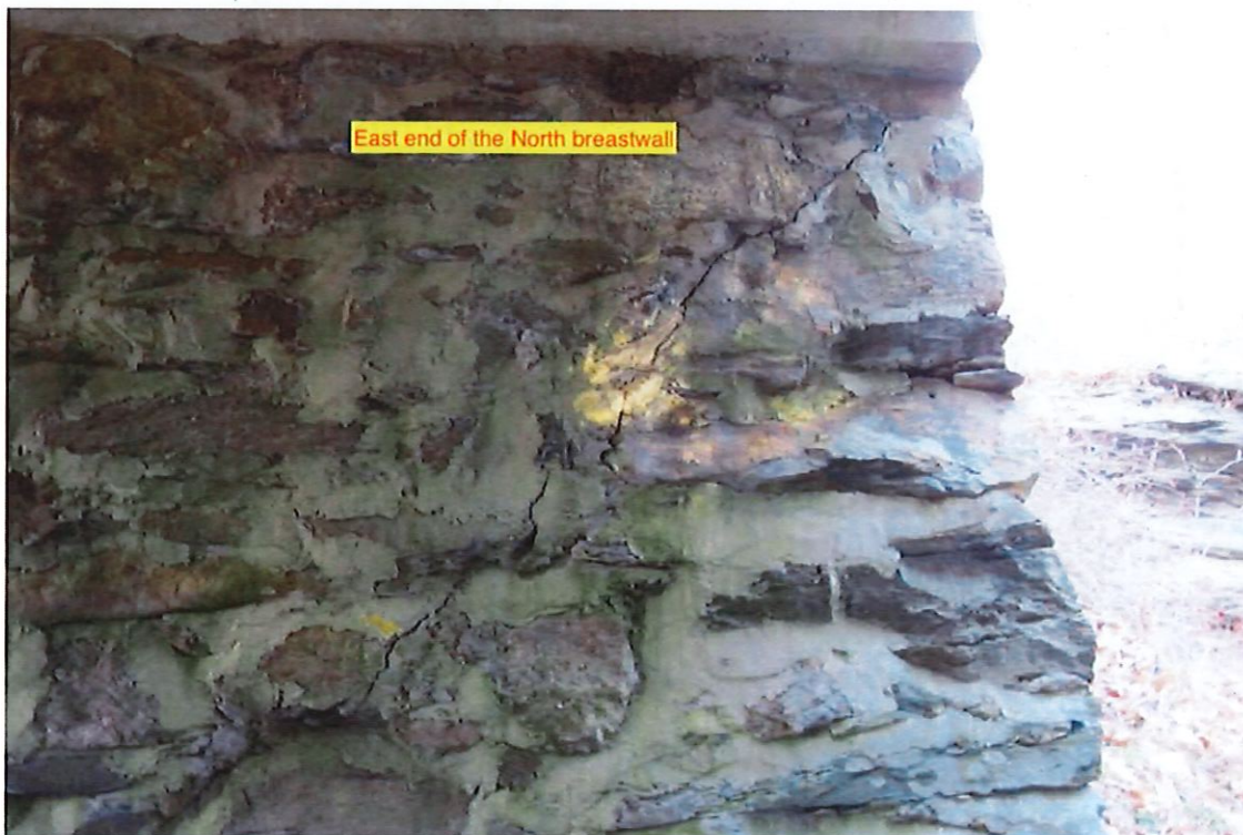
Photo 6: Crack to the East end of the North breastwall.
