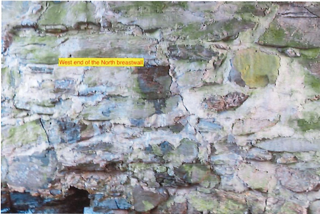
Photo 5: Crack to the West end of the North breastwall.
