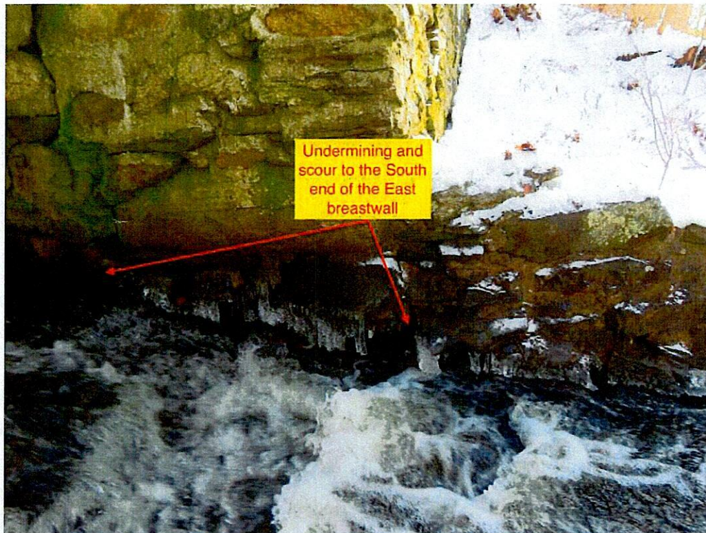
Photo 9: Undermining and scour to the South end of the East breastwall.
