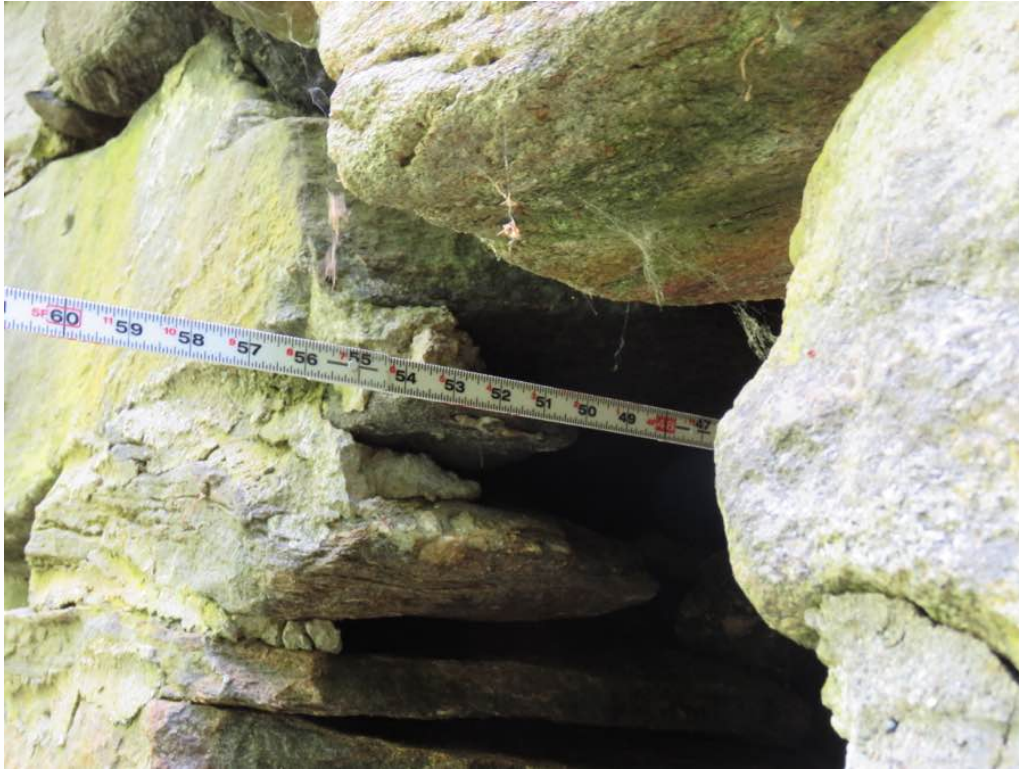
Photo 9: Penetration to the void on the Southwest wingwall.
