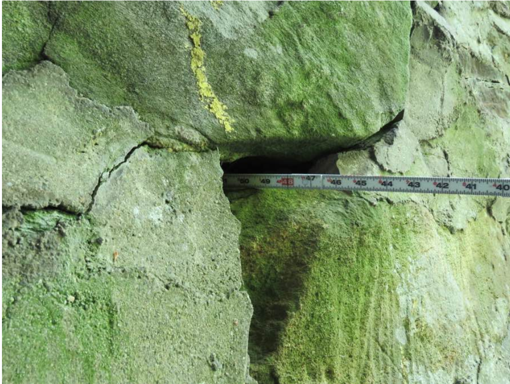
Photo 3: South breastwall, West end showing penetration.
