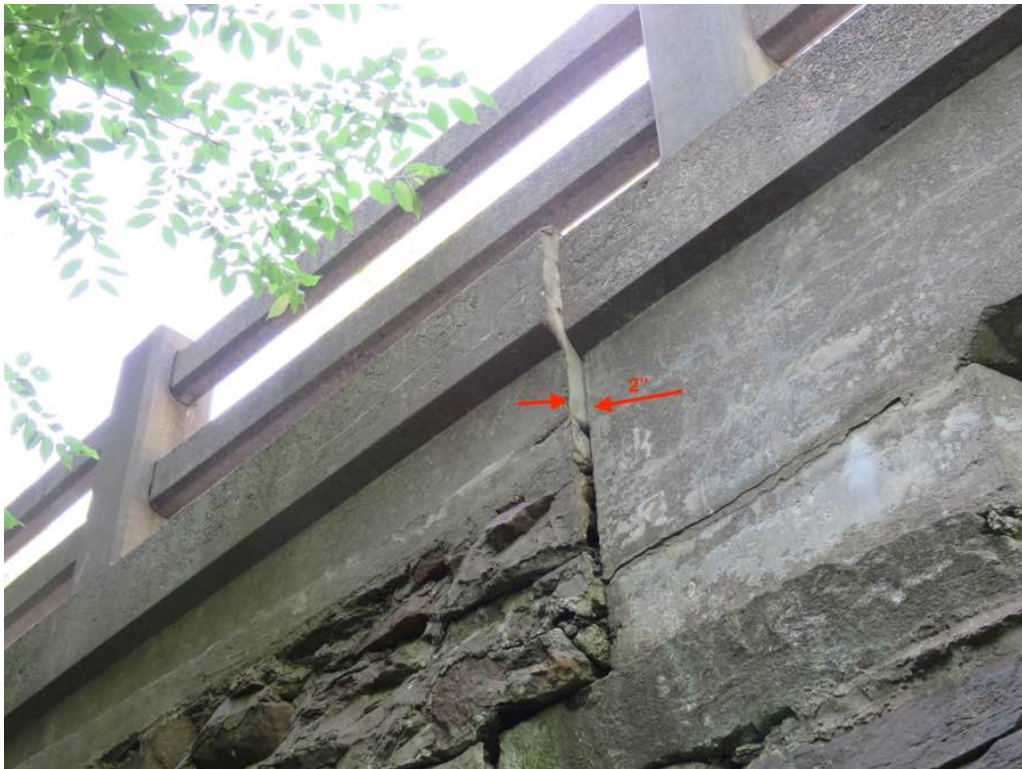
Photo 14: Southeast wingwall displacement.
