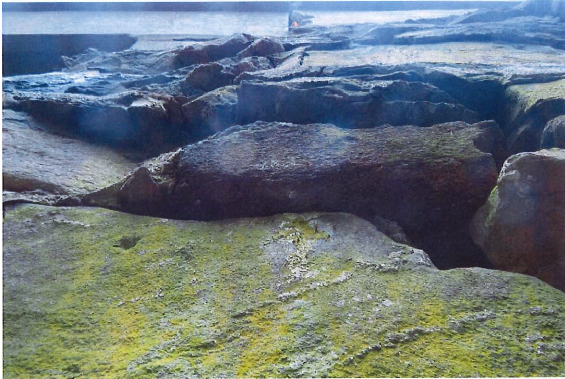
Photo 6: Southwest wingwall, outward displacement locus closeup.
