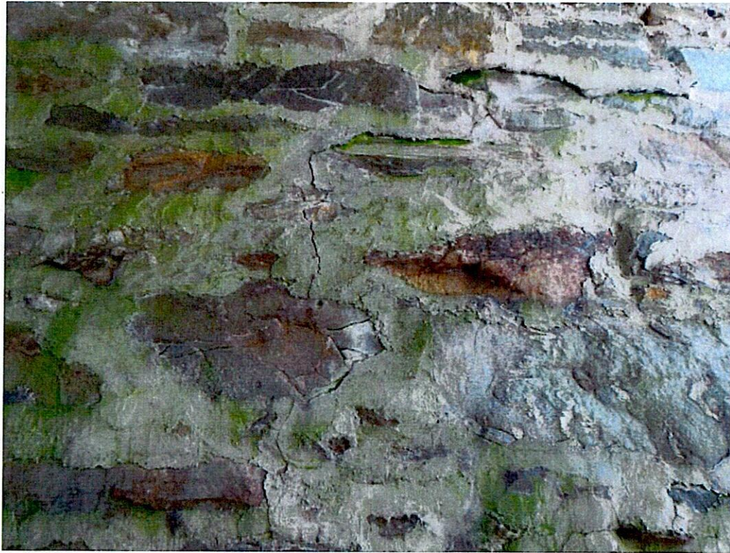
Photo 5: Cracked stone and pointing at the East breastwall near South end.
