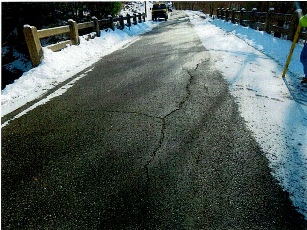
Photo 4: Cracks to the West approach pavement.
