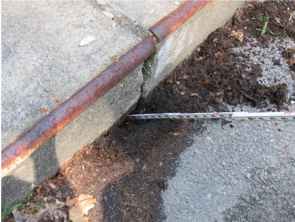
Photo 13: Hole at the joint interface.
