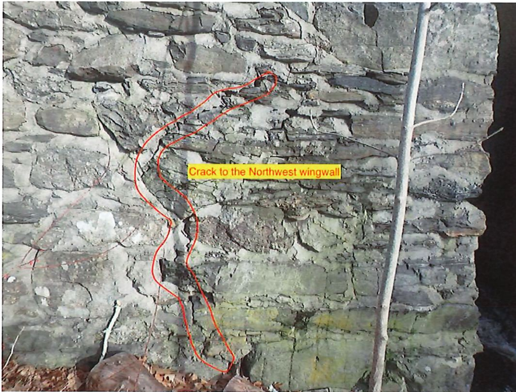
Photo 13: Northwest wingwall displacement and crack.
