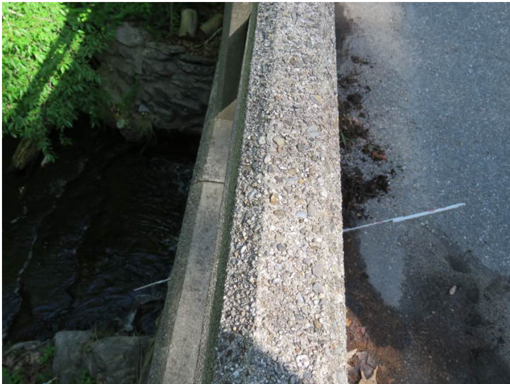
Photo 12: Hole at the interface joint.
