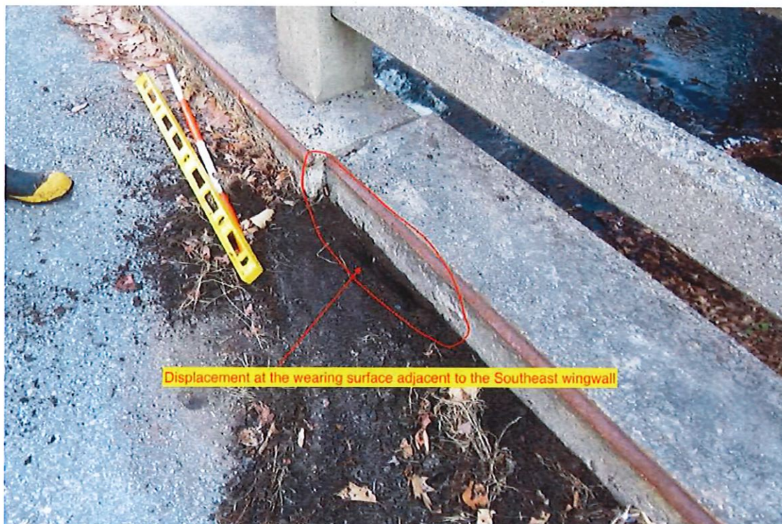
Photo 12: Displacement to the Southeast wingwall at the top.
