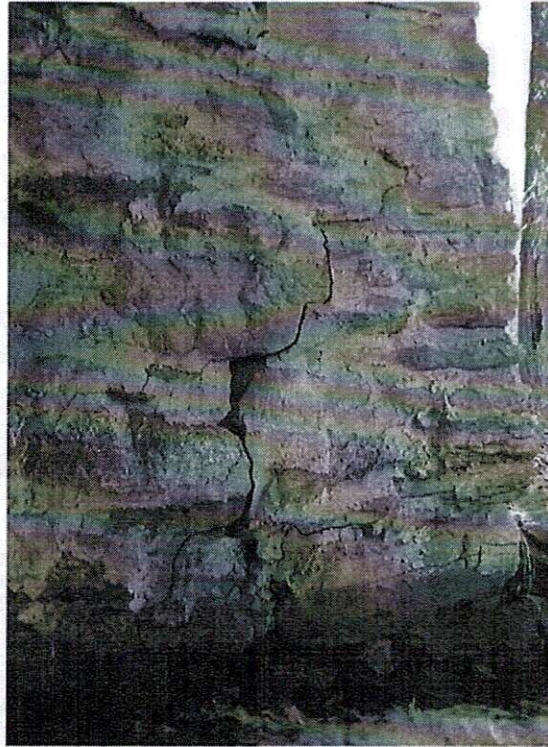
Photo 1: South breastwall, west end crack.
