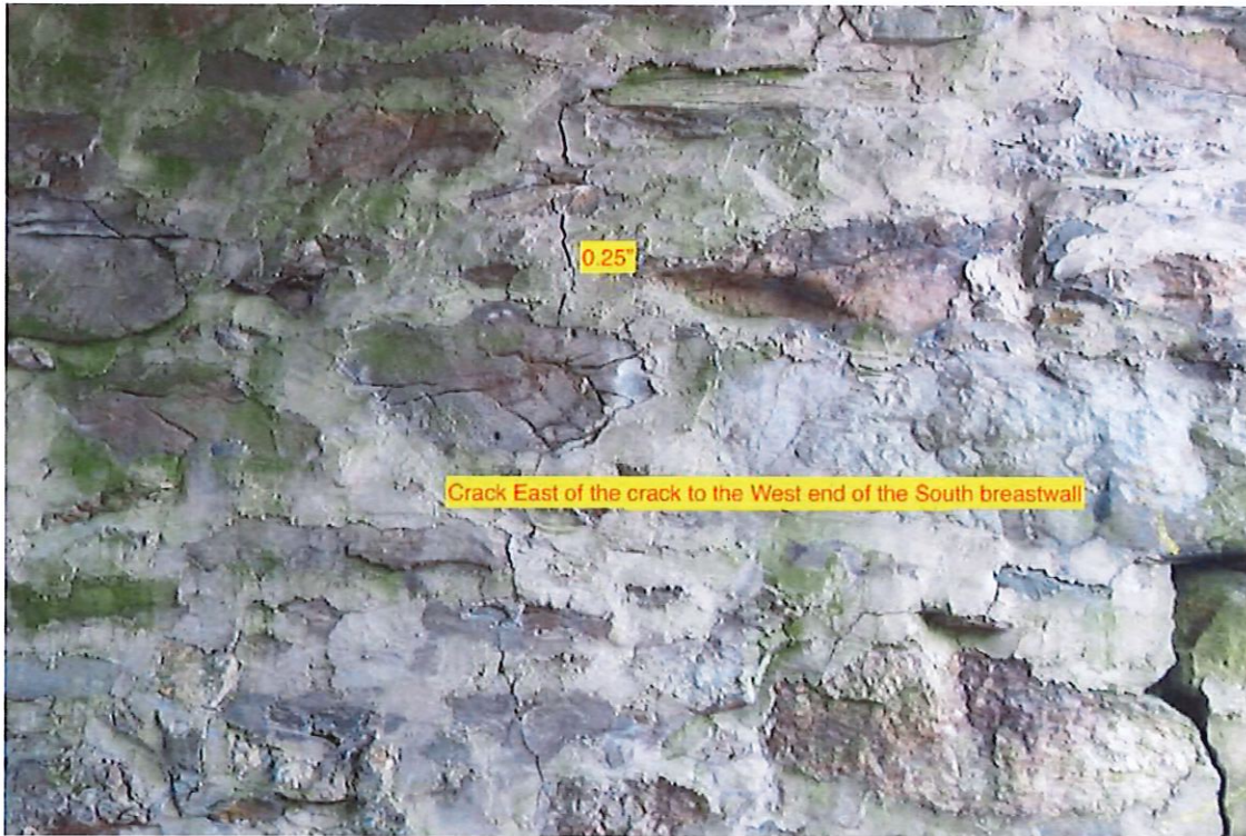
Photo 3: Crack to the South breastwall.
