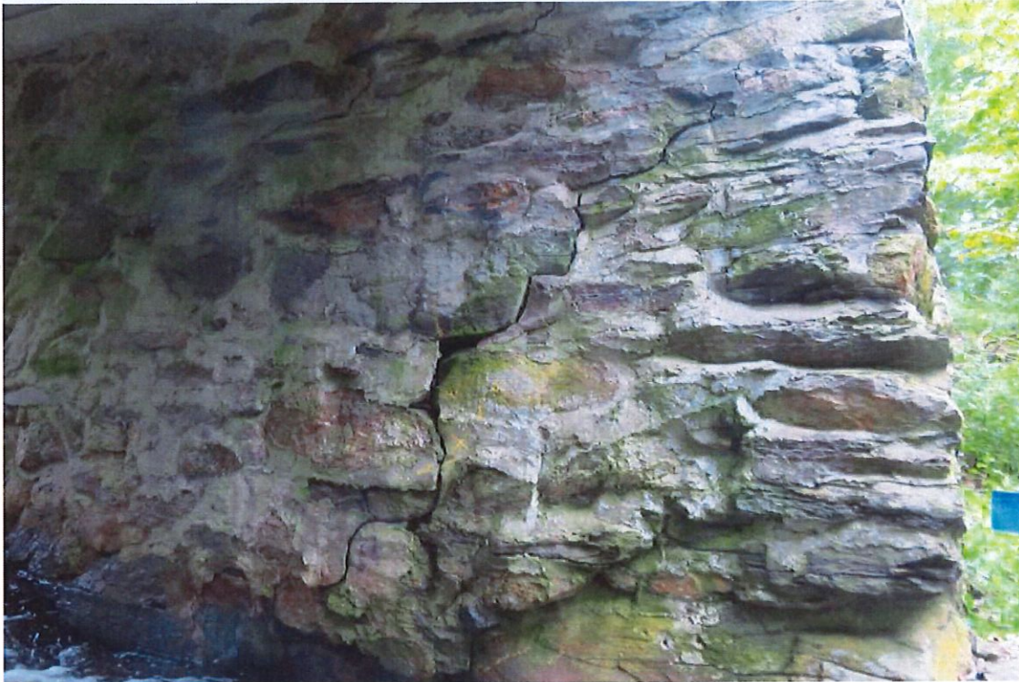
Photo 1: South breastwall, west end crack.
