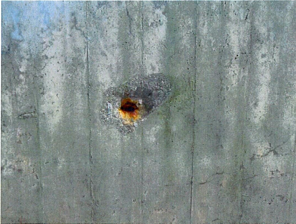
Photo 1: Spall to the North end of the deck slab.
