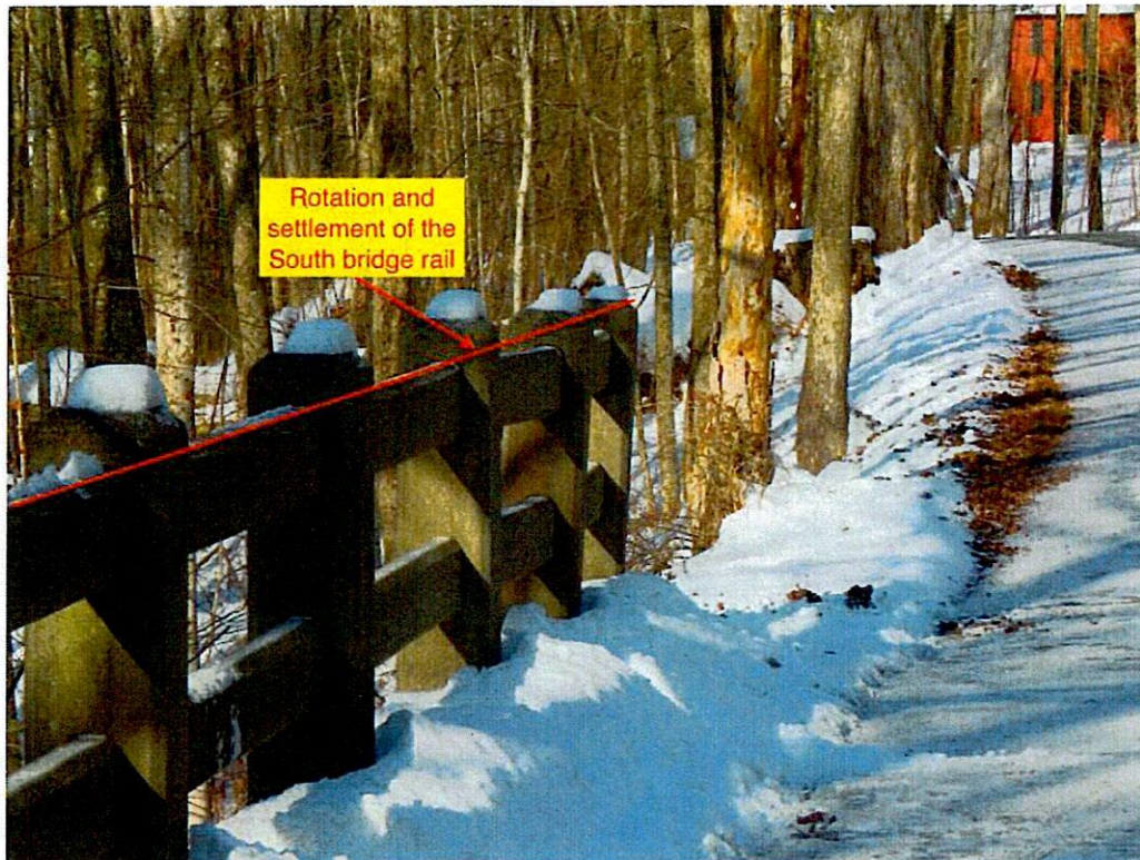
Photo 3: Rotation and settlement of the Southwest approach rail.
