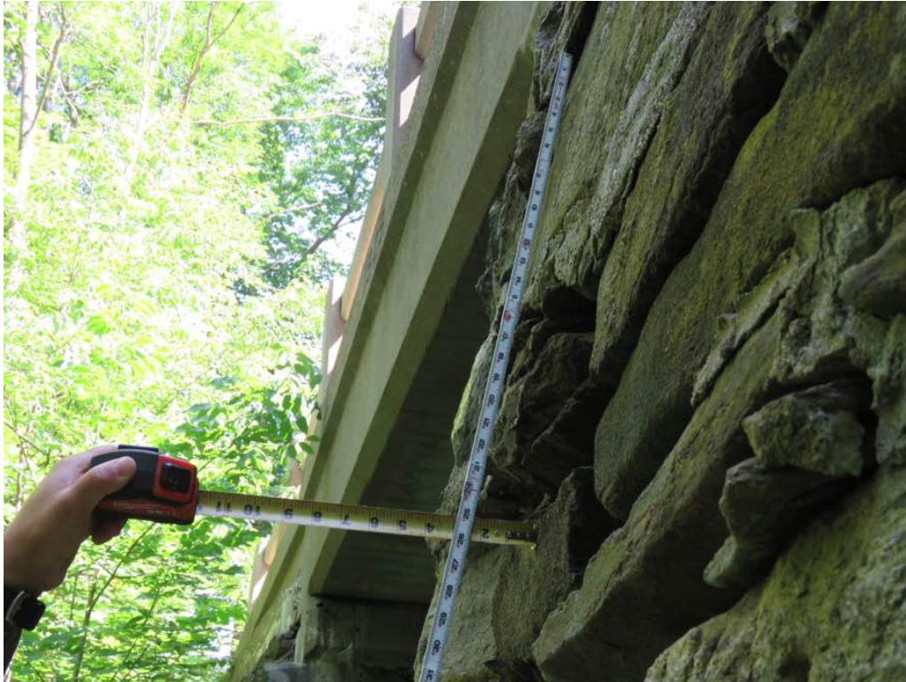
Photo 11: Outward displacement measurement to the Southwest wingwall.
