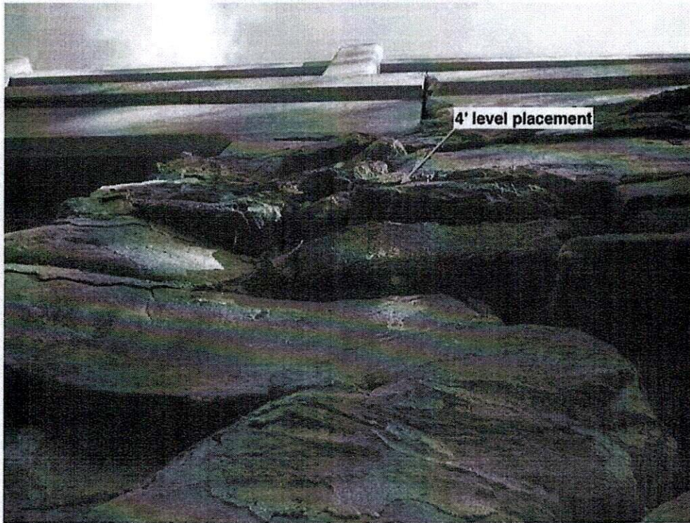
Photo 6: Southwest wingwall, outward displacement locus closeup.
