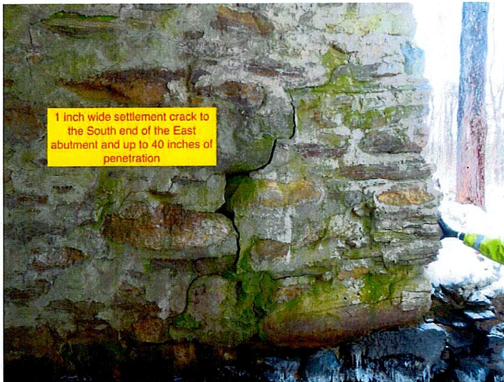
Photo 7: Settlement crack to the East breastwall at the South end.
