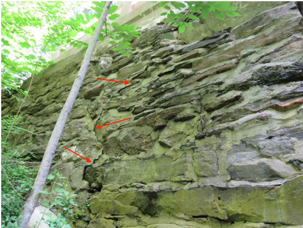
Photo 16: Northwest wingwall cracks.
