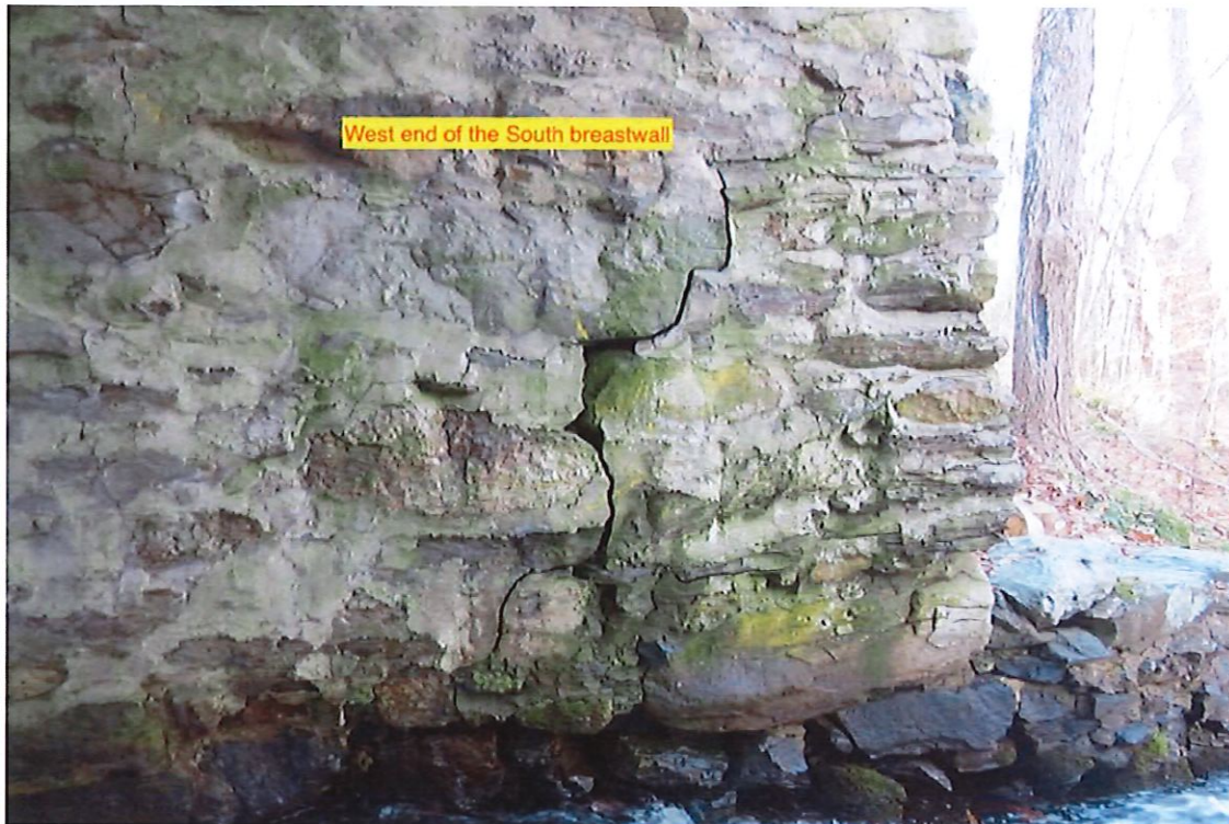
Photo 1: Crack to the West end of the South breastwall.
