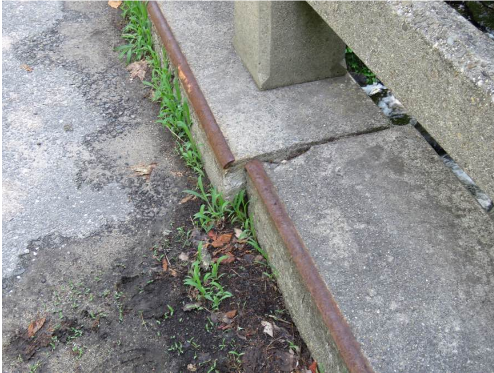
Photo 15: Southeast wingwall displacement to the top.
