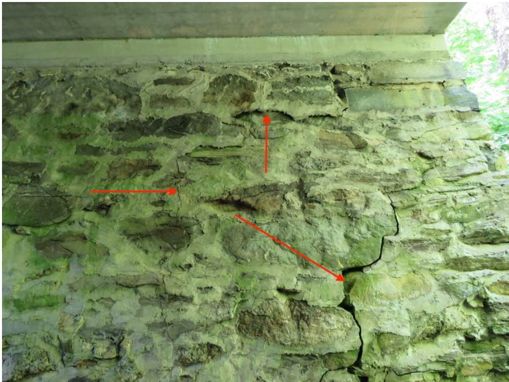
Photo 2: South breastwall, West end showing cracks.
