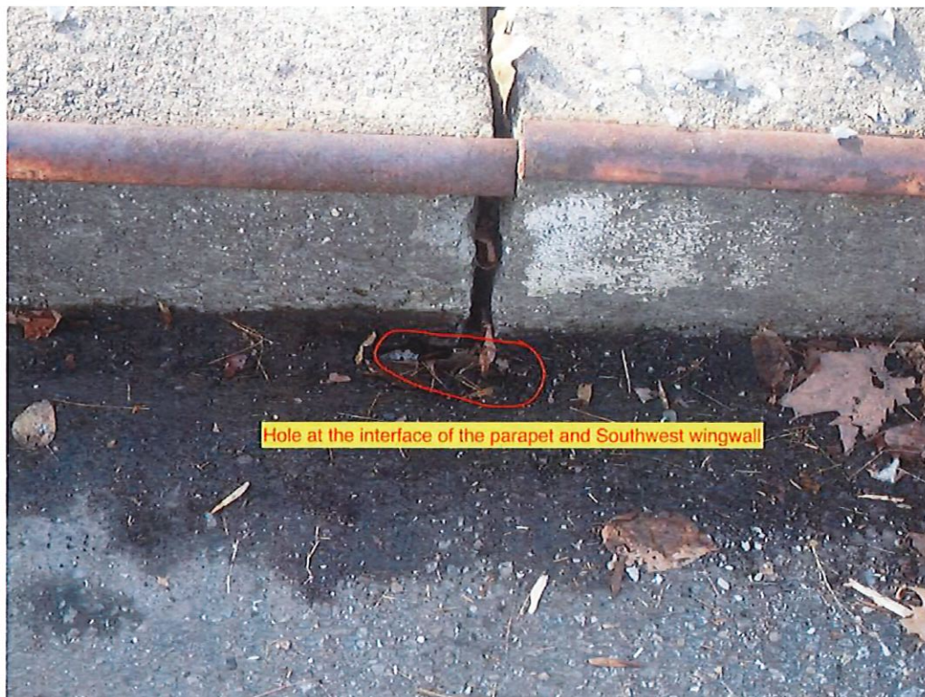
Photo 10: Hole at the wearing surface and the Southwest wingwall.
