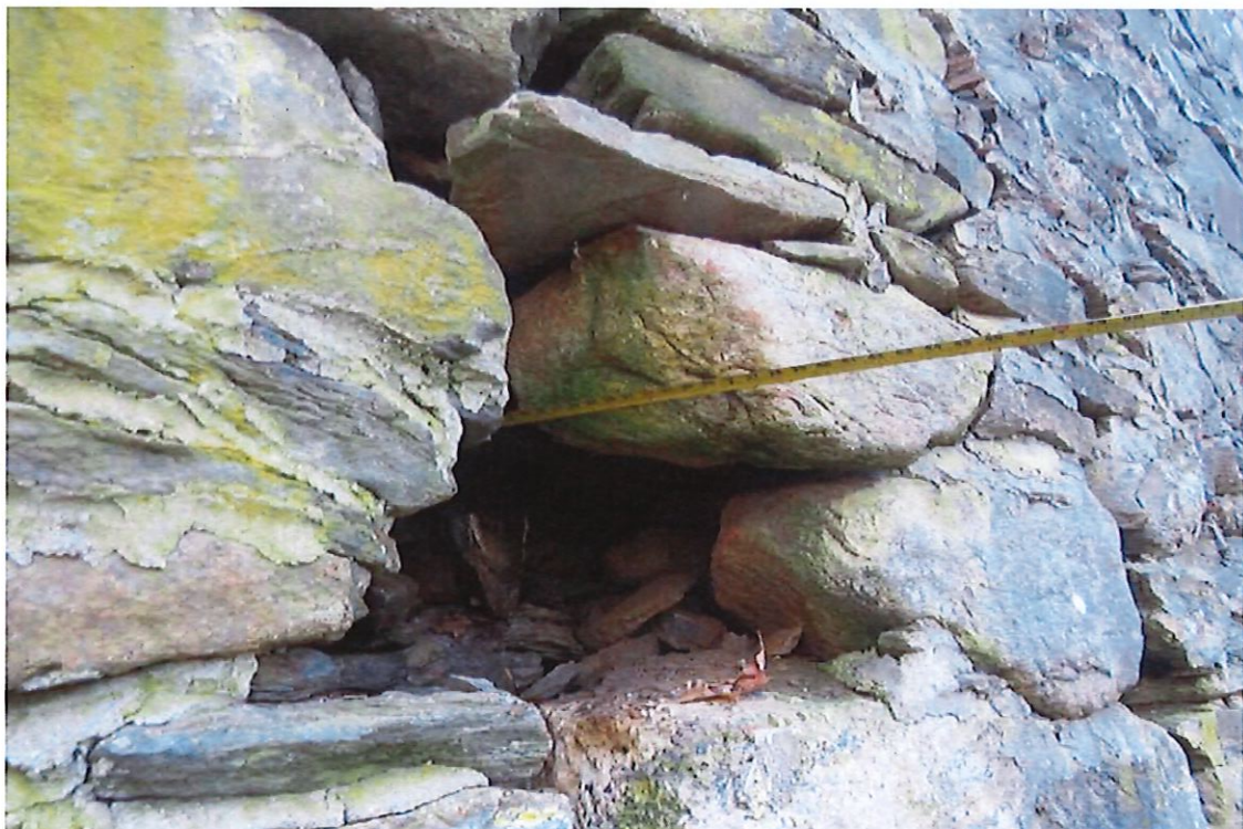
Photo 8: Area of missing stones and void to the Southwest wingwall.
