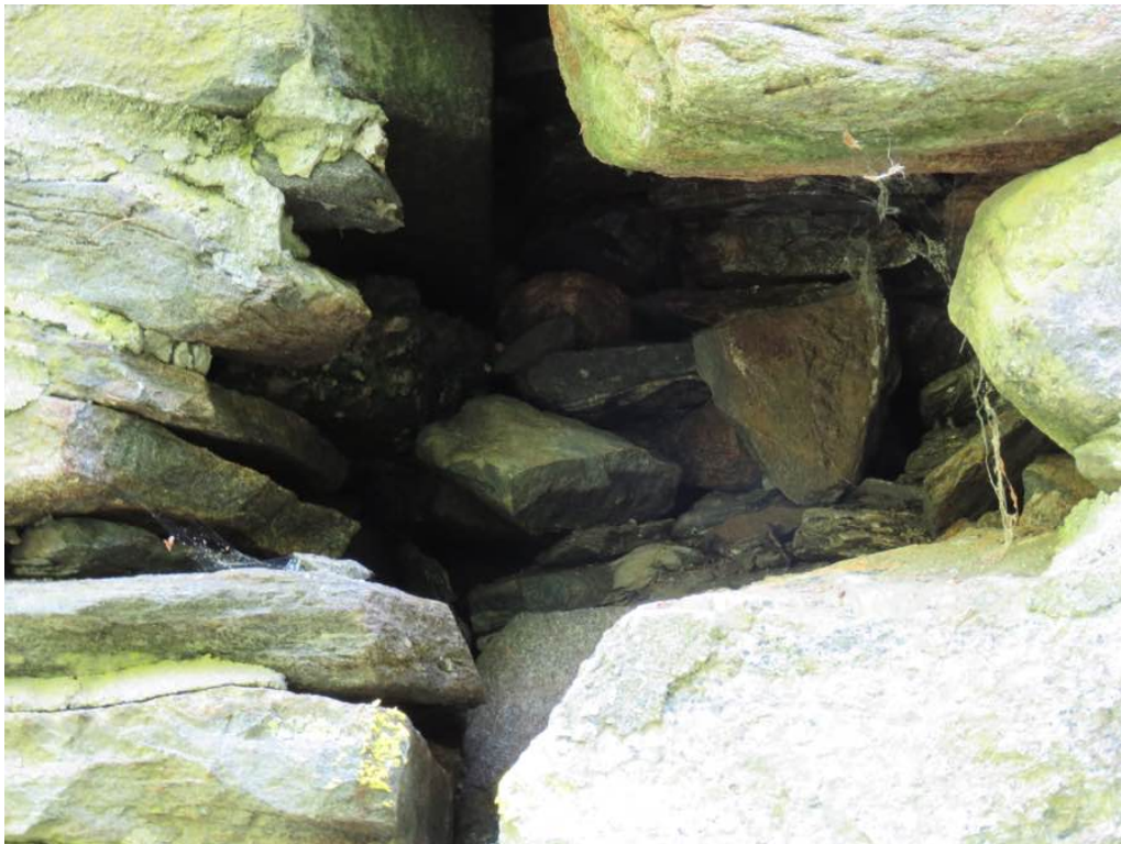
Photo 10: New loss of backfill and stones in the void.
