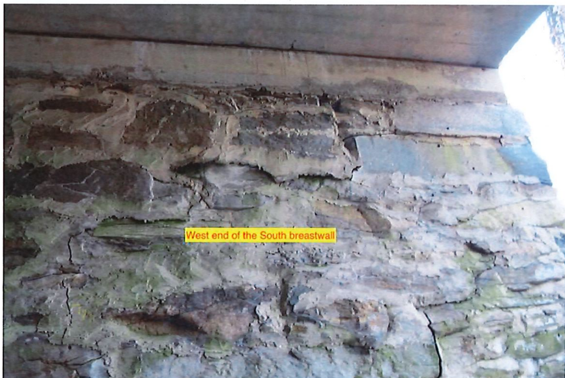
Photo 2: Cracking at the top of the South breastwall at the West end.
