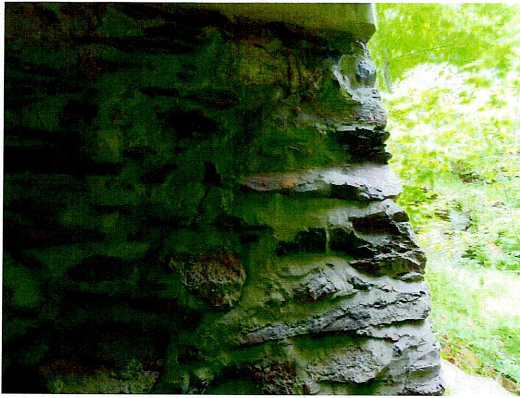
Photo 1: Cracking to the pointing at the Northeast corner.
