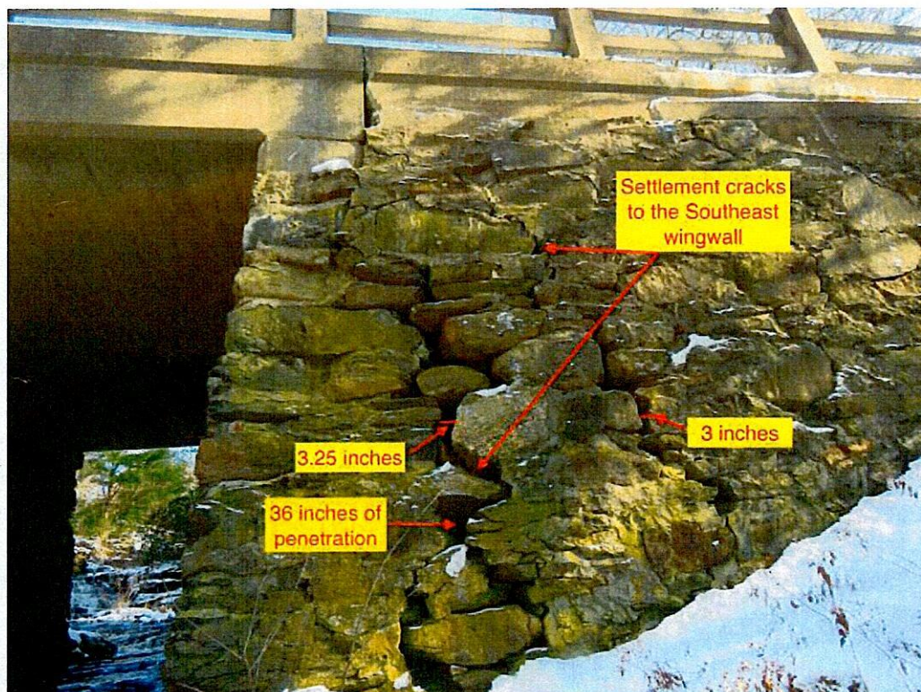
Photo 10: Large settlement cracks to the Southeast wingwall.
