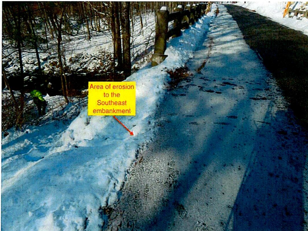
Photo 12: Area of erosion to the Southeast embankment.
