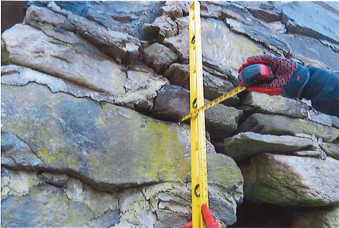
Photo 9: Outward displacement to the Southwest wingwall.
