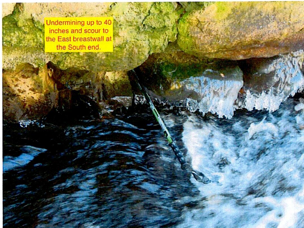
Photo 8: Undermining and scour to the South end of the East breastwall.
