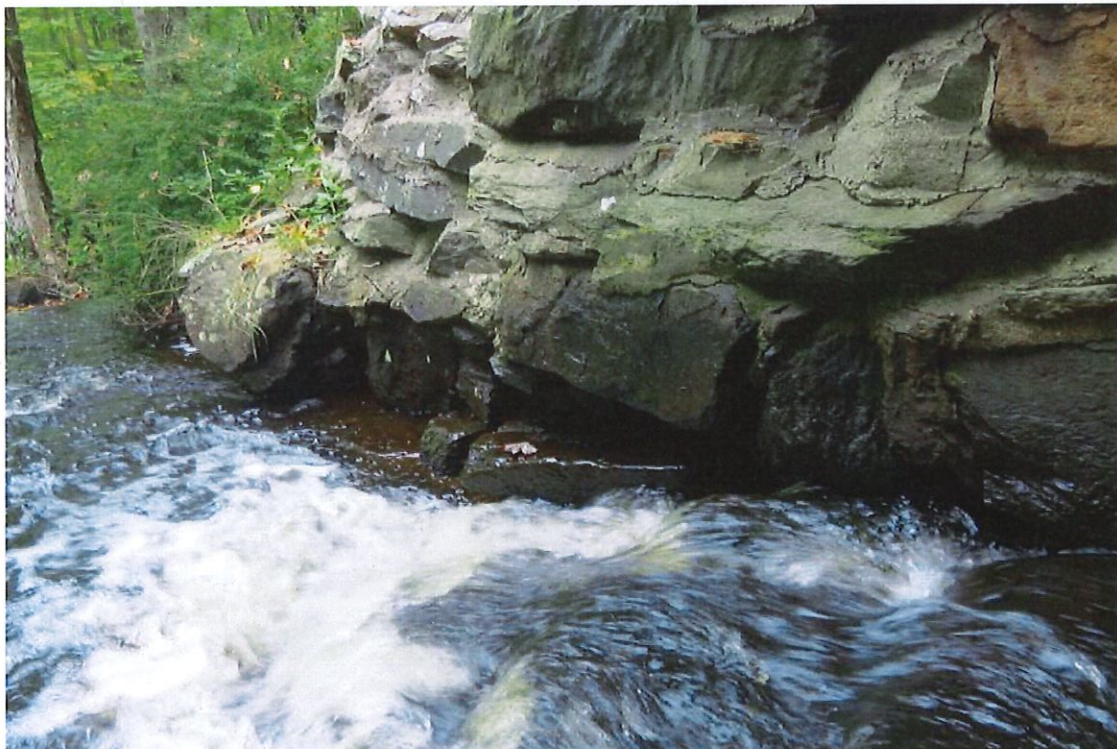
Photo 4: North breastwall, west end bottom gap in masonry.
